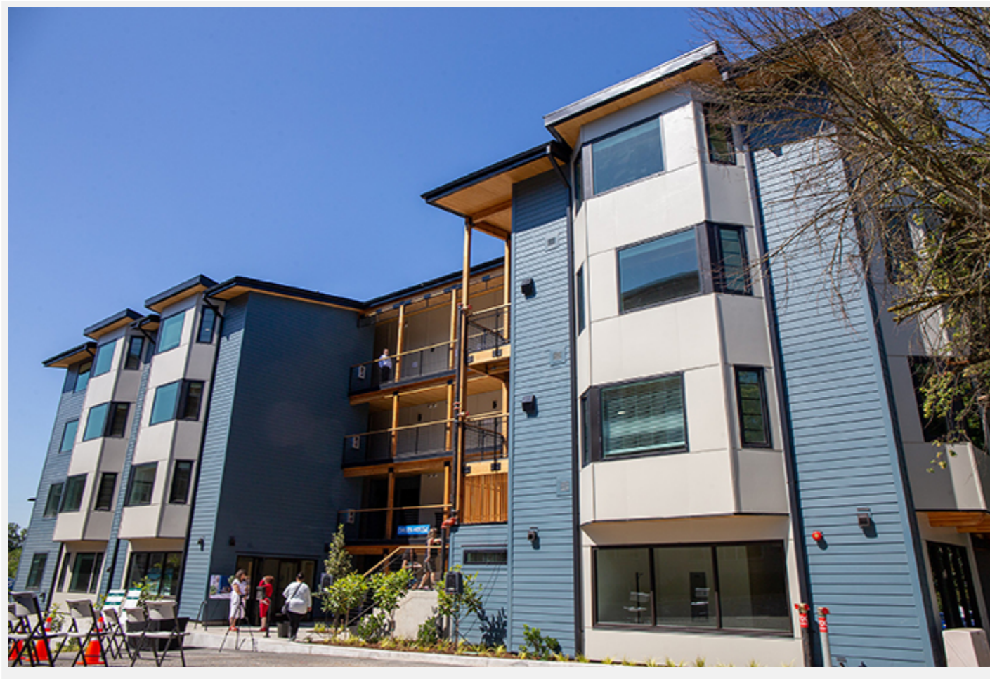
The Chiles House is located near the Catholic Charities of Oregon headquarters in Portland at 2740 S.E. Powell Blvd. (Alex Jensen/DJC)
